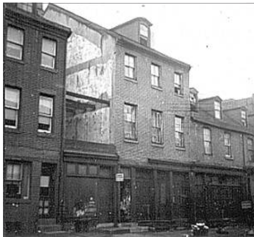
18th-century buildings in dilapidated condition. 217 Pine Street, December 1946.
